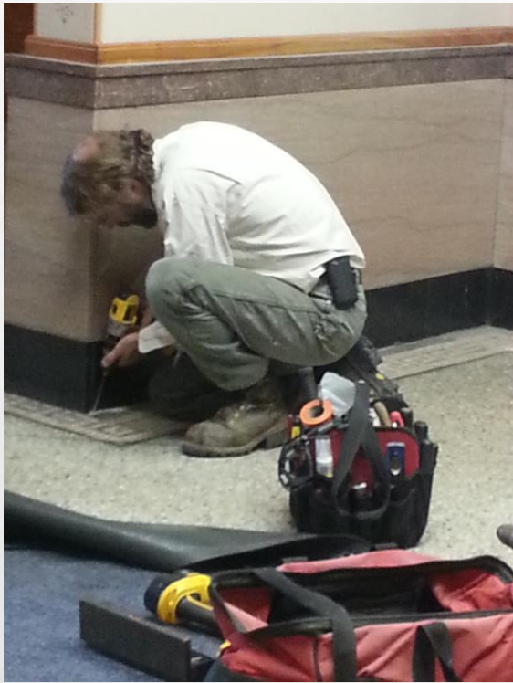
Marc Aucoin, Electrician & knower of all the TFL nooks & crannies
