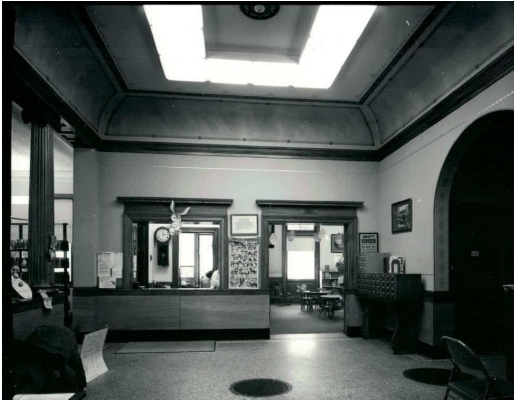
Image 68, First Floor Lobby (now circulation area) facing west, photo taken by: Ernest Gould, 4/6/1990.
