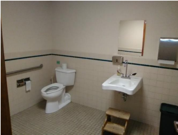
Image 101, Existing lower level ADA restroom
