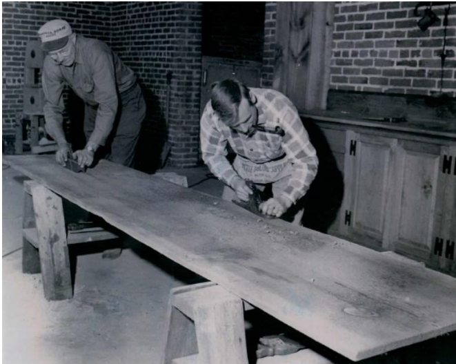
Image 5. Forrest and Archie Morse in 1970 building cabinetry. Source unknown.
