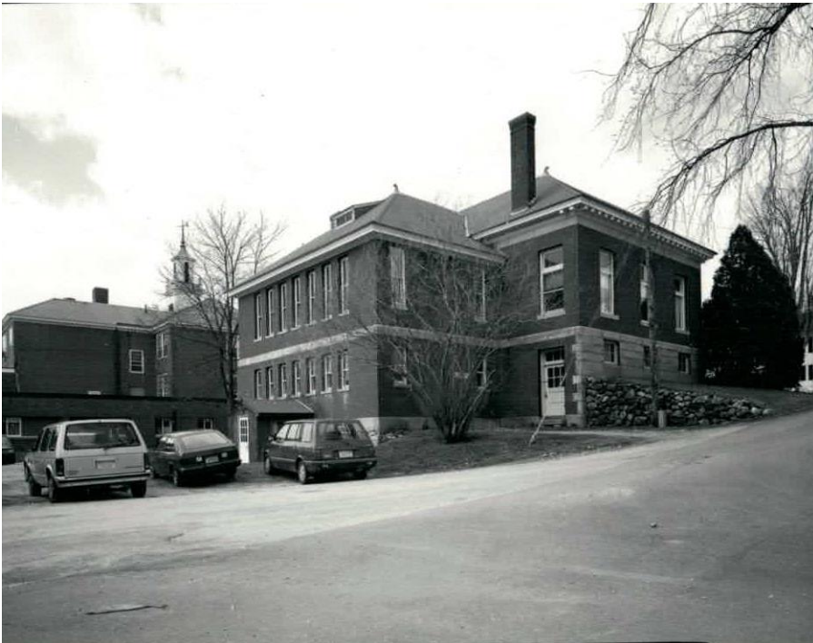
Image 20, Back view from south east Location, photo taken by: Ernest Gould, 4/6/1990.
