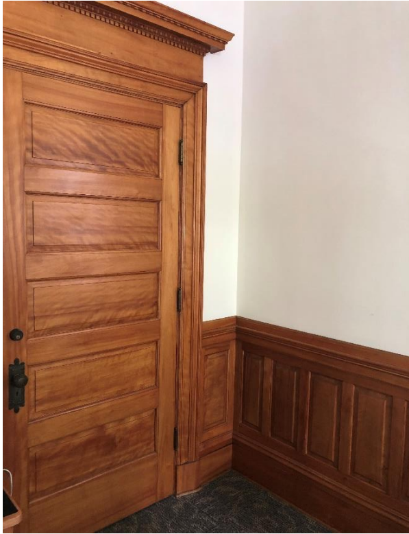
Image 50, An example of the 5-panel doors, hardware and wood wainscoting at the non-fiction room and NH Room, photo taken: 6/11/2020.
