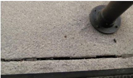
Image 75, Gap in granite at south entry
