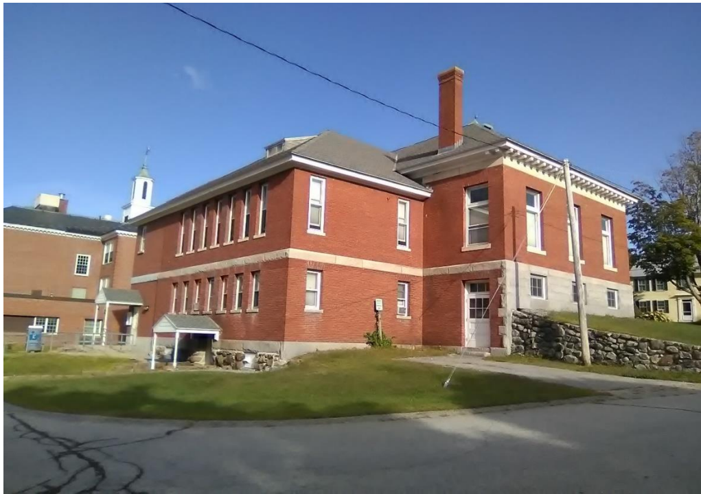
Image 13. South east elevation. Notice the corner quoins and how the dentil ends. Facing west, photo taken: 10/2019.
