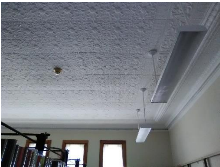
Image 94, Tin ceiling with pendant florescent lighting fixtures
