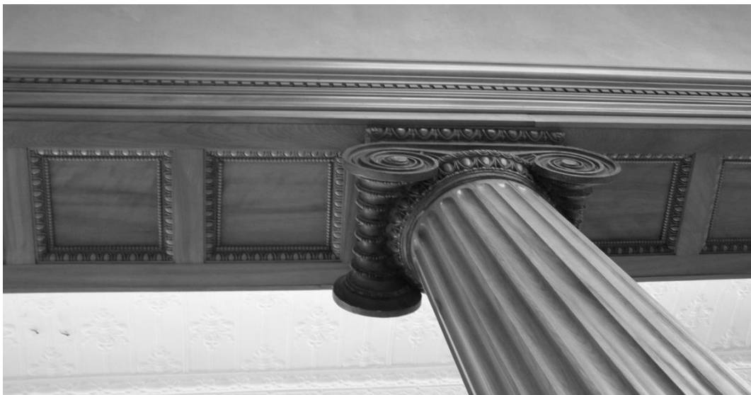
Image 49, One of the four columns on the Main Floor, this photo shows the intricately detailed column in the receiving area, facing south, photo taken: 1/31/13.
