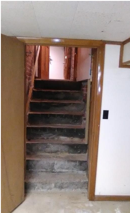
Image 89, Sub-basement stair to J-room
