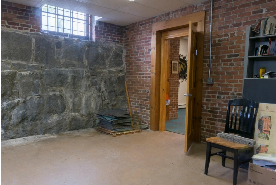
Image 54, Basement Archives (now storage outside of mechanical room), facing west, photo by: Joshua Colby, 4/22/2019.
