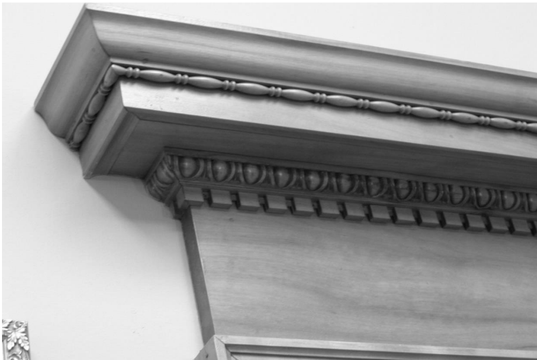
Image 51, Door casing detail, photo taken: 1/31/13.
