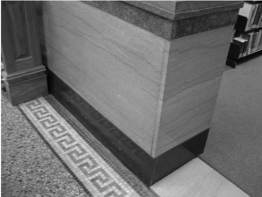
Image 52, Marble wainscoting at the room dividers and thresholds. Note the Greek Fret and terrazzo floor, face south east. photo taken: 1/31/13
