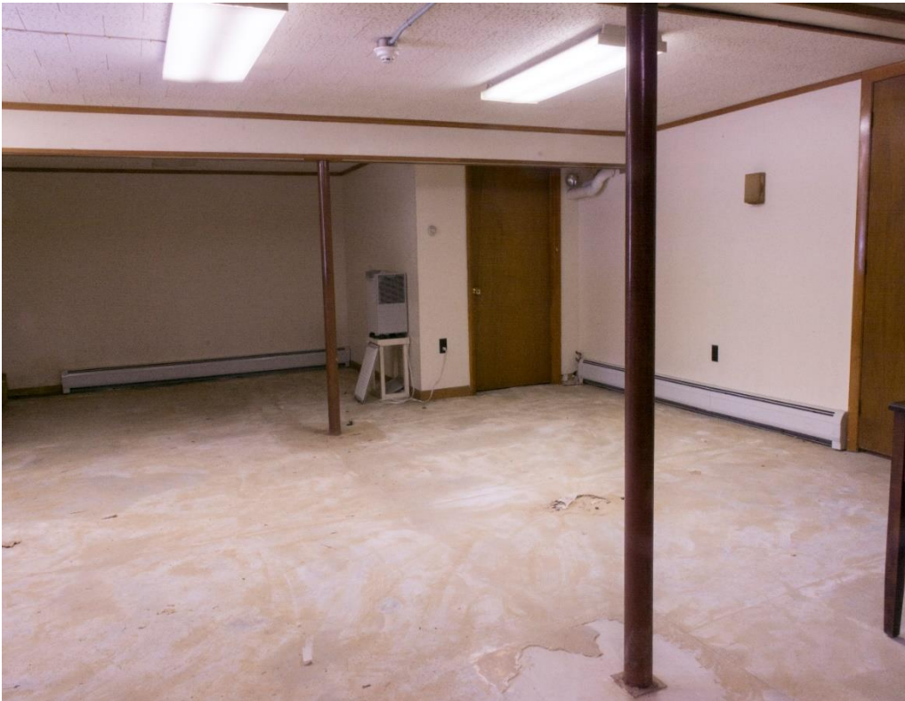
Image 67, Sub-basement (now vacant) facing west, photo taken by: Joshua Colby, 4/22/2019.
